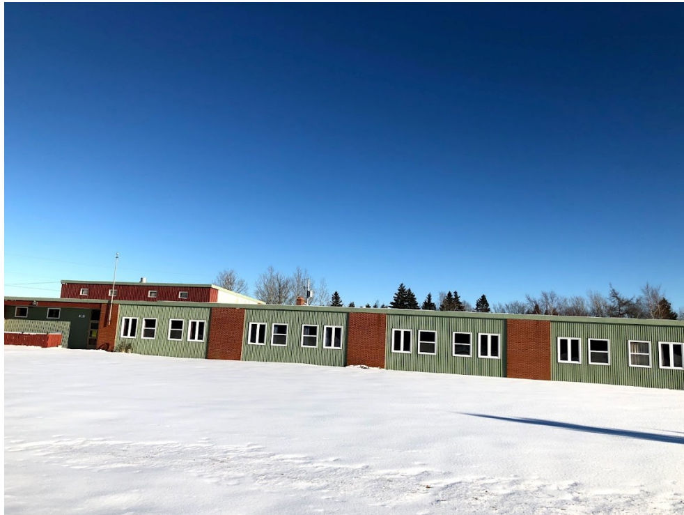
Figure 10. The former Maitland District Elementary School, February 2021
