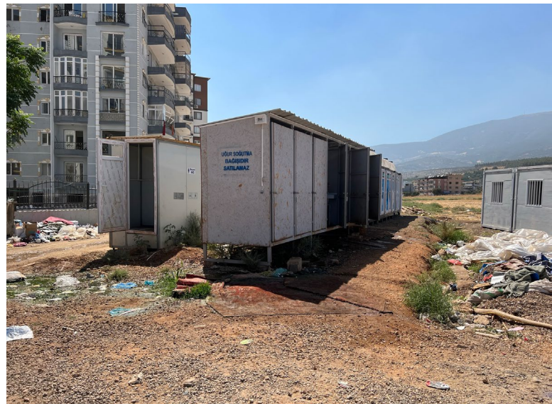
Figure 30. Washroom facilities in front of the adjacent building; septic connections from adjacent buildings are above ground.
