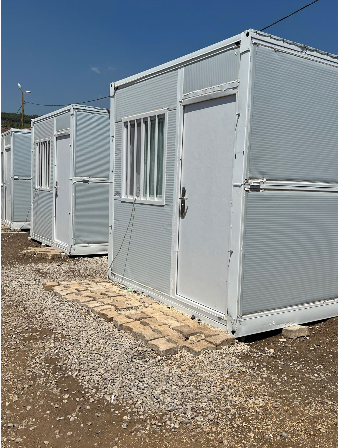
Figure 39. An inhabited container that shows that there is no infrastructure needed for the structural stability when placing the containers on ground. Most containers are lifted using blocks to eliminate direct contact with ground to prevent water from getting into the container.
