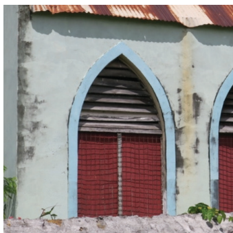
Louvred window on the existing building (Bailey 2023)
