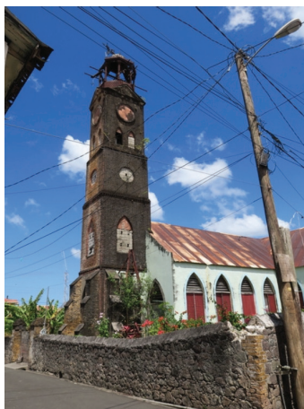
The existing steeple (Bailey 2023)
