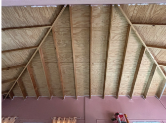
Exposed roof structure in a residential home
