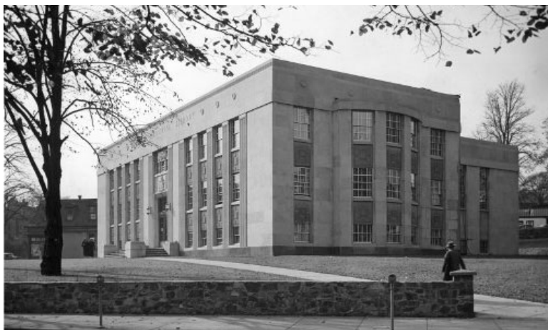
Exterior of the library after completion 1951 (Halifax Military Heritage Preservation Society n.d.).
