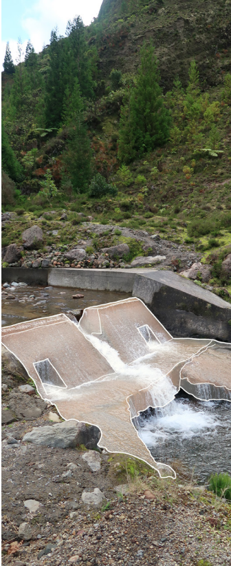
The hydroelectric dam in the Valley of Lombadas.
