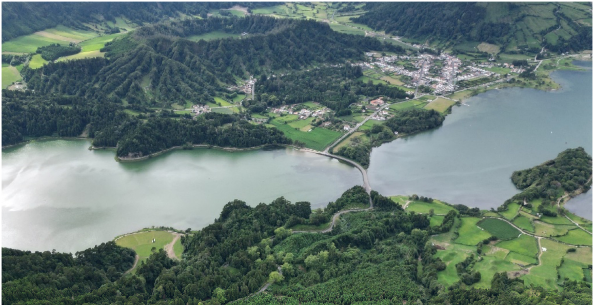
Lagoa das Sete Cidades reflecting the two colours. The Ponte dos Regos bridge runs across the area between the “two” lakes.
