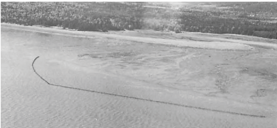
Weir at Economy point at Minas Basin (photo from Gordon 1993, 55).
