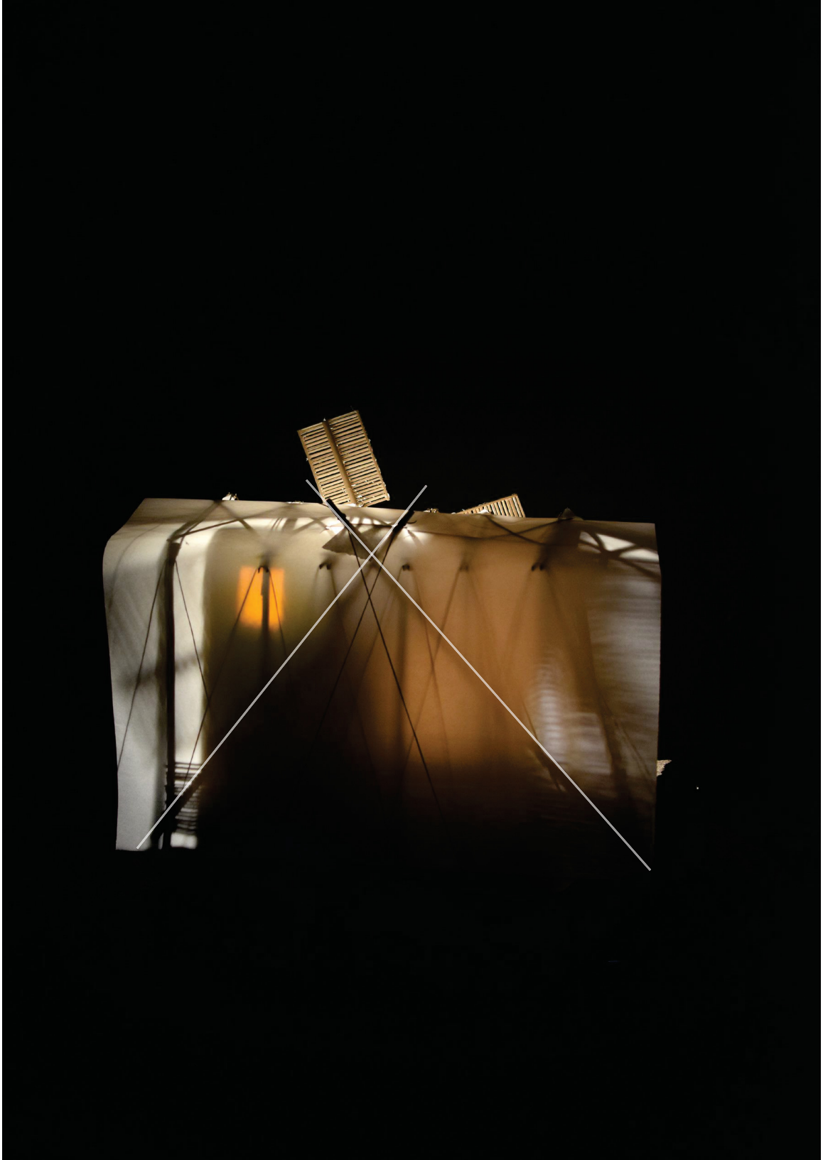
The roundwood cross-bracing eliminates the need for structural support from the screen-wall, creating an opening through which the yellow light can travel and project onto the veil.
