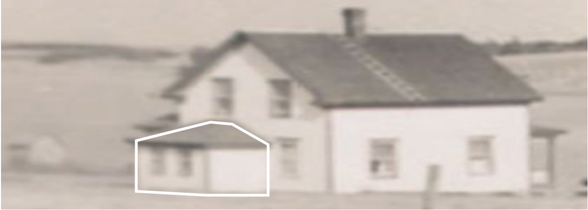
Vernacular saddlebag (“bump”), typical in Acadian houses and farmhouses, reimagined as a totemic element that facilitates embodied architectural experiences (based photo from Nova Scotia Archives 1951).
