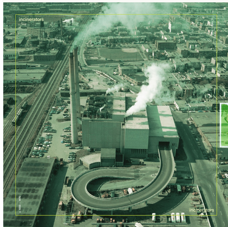
Information: Diagram of incinerator by author. Photograph of Des Carrières Incinerator in Rosemont, Montréal (Fonds des affaires institutionnelles1974).
