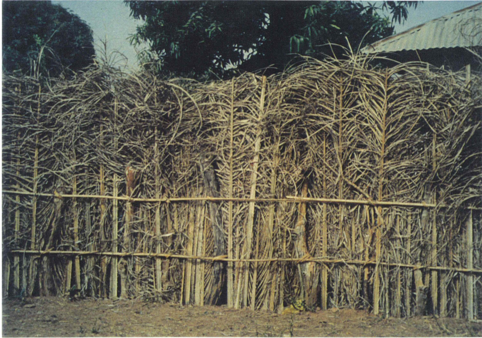
Figure 4a: Compound exterior wall using palm fronds as construction material.
