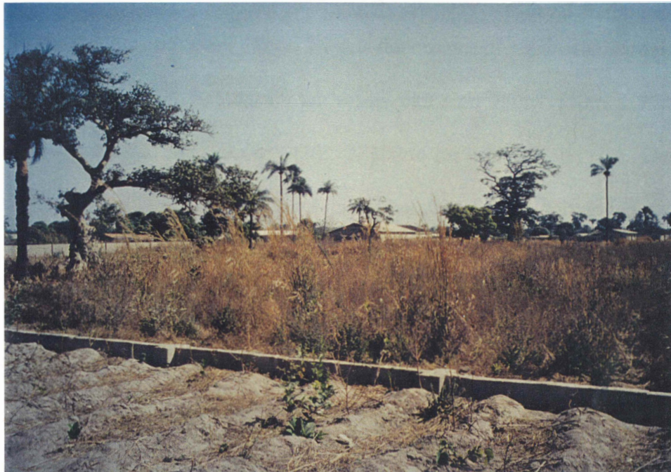
Figure 3b: Typical urban compound exterior wall incomplete with footing only that delineates the plot boundary.
