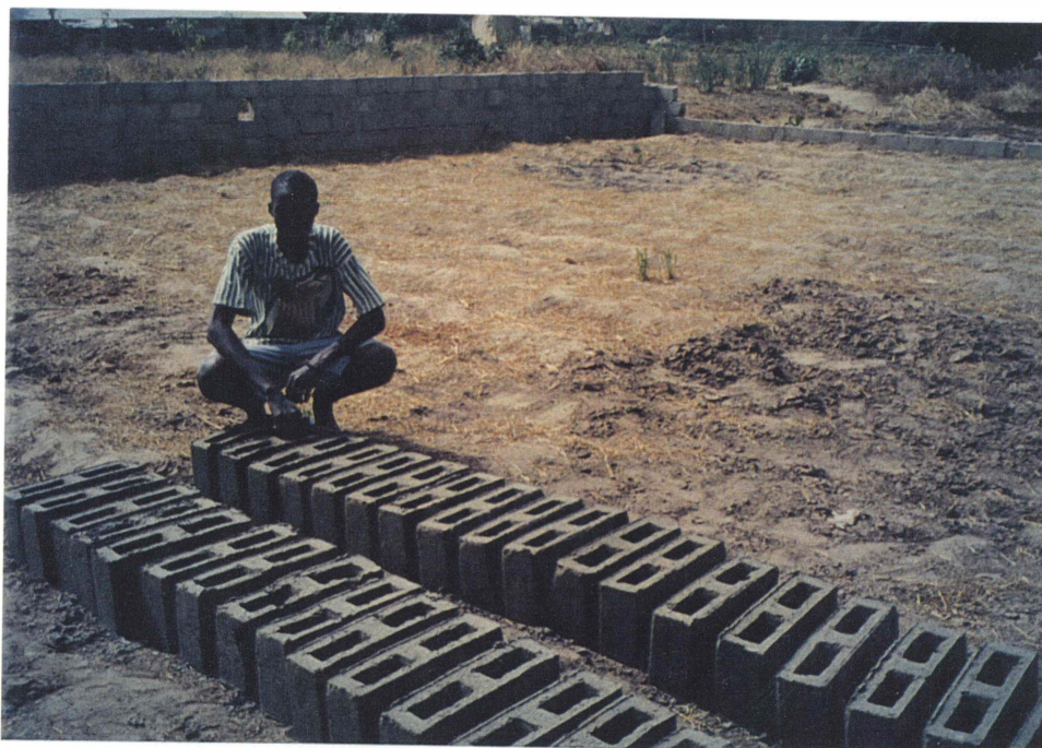
Figure 7b: Concrete blocks which are formed on site are used for wall and house construction.
