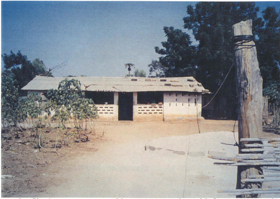
Figure 8a: Single story compound house construction with front outer porch and metal roof.
