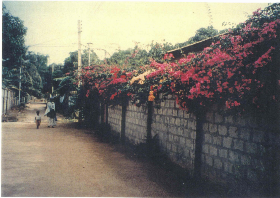
Figure 3a: Typical urban compound exterior wall completed with concrete blocks.
