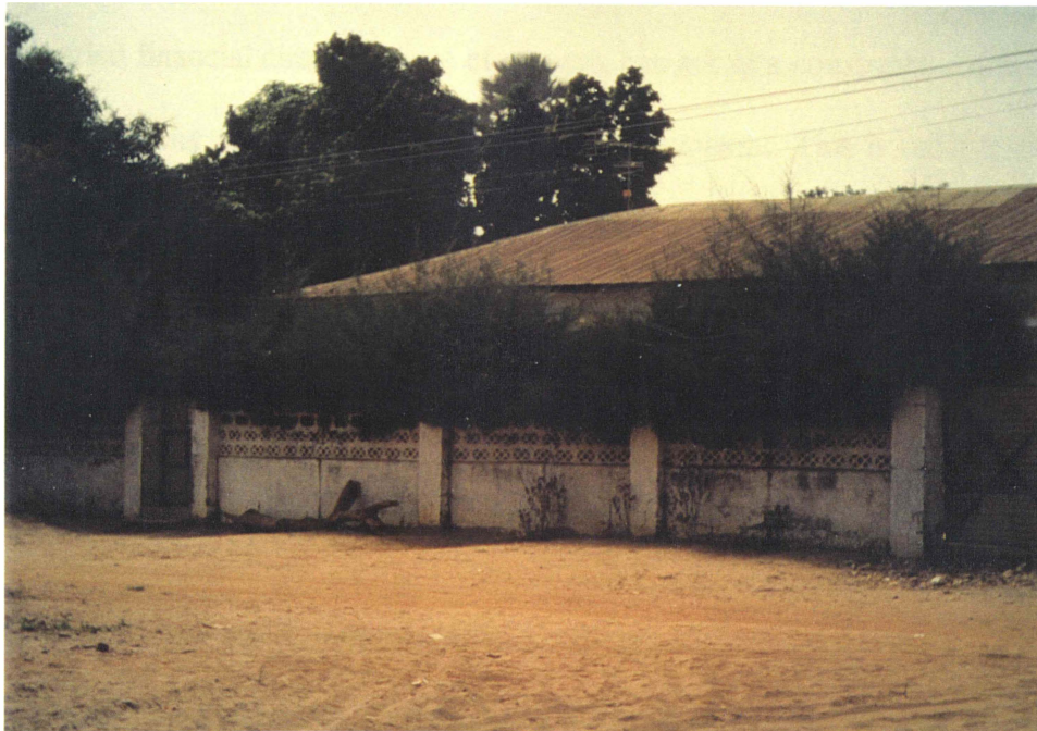
Figure 11b: Compound exterior wall incorporating both block work and vegetative materials.
