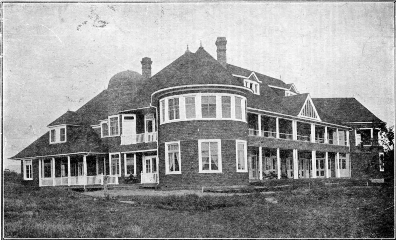
The one-building Provincial Sanatorium as it was in 1910 when Dr. Miller took charge. After many alterations and adaptations it continues in use today as the Annex, devoted to the care of children on the first floor and convalescent women on the second floor.
