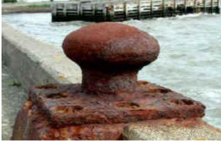
Figure 3 - Uniform corrosion [5]
