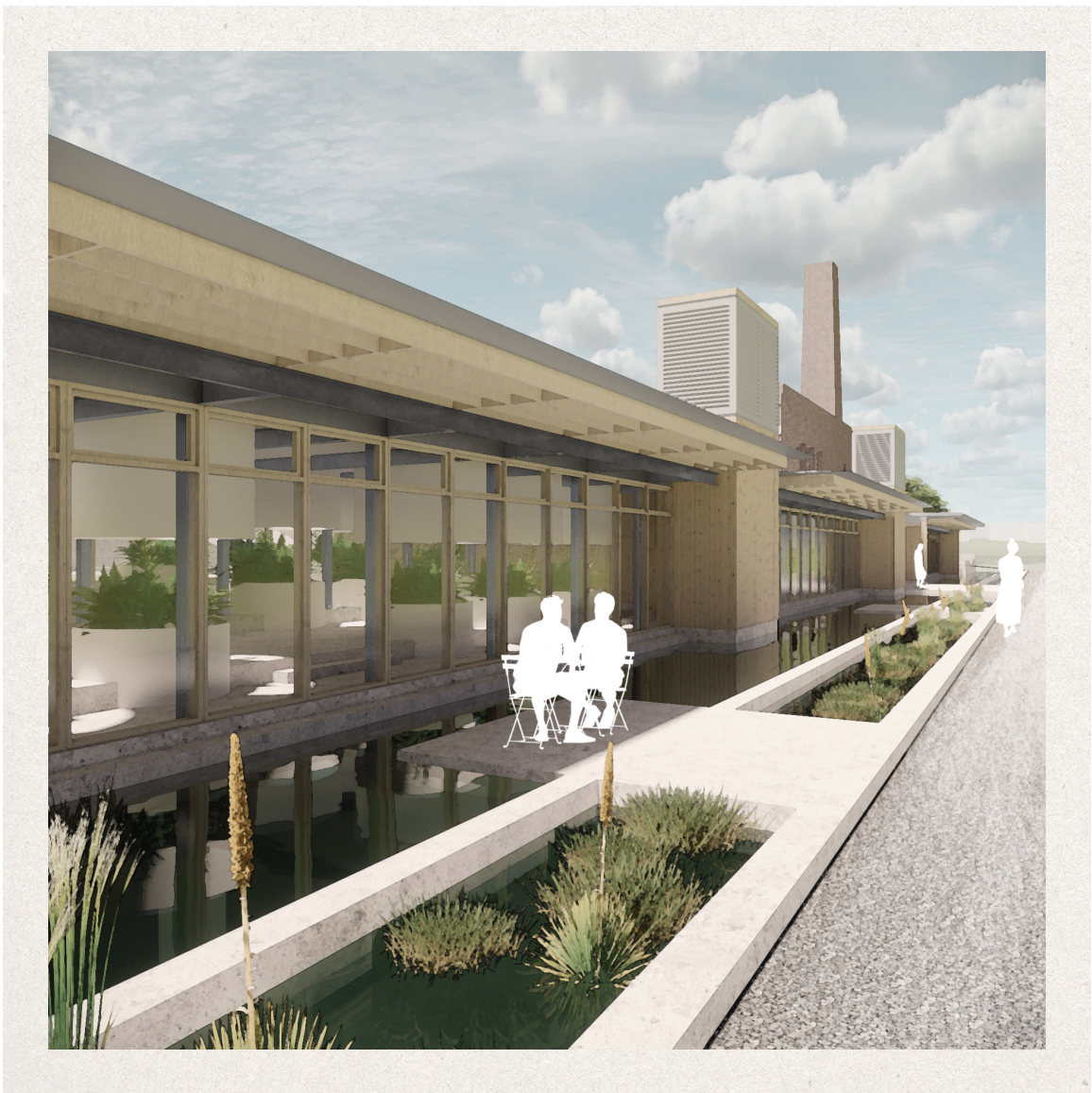
Solar Aquatics area of the Powerhouse Extension. Structural load-bearing walls and totemic wind catchers clad in wood siding and metal vents act as stereotomic elements of the extension.
