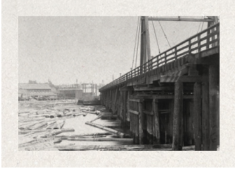
Photograph of Rock Bay Bridge (Helmcken 1912)
