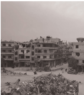
Figure 40. Rubble-filled areas in Harasta (“Dron Footage: Syrian Government Rehabilitates Liberated Harasta City” 2018)
