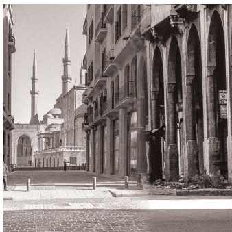
Figure 12. Post-war rebuilding efforts in Beirut (Kozlova 2023)
