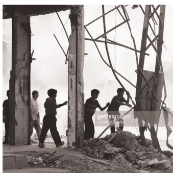
Figure 25. Syrian children play amid the rubble of destroyed buildings being remove by a bulldozer in Harasta. (Beshara 2018)
