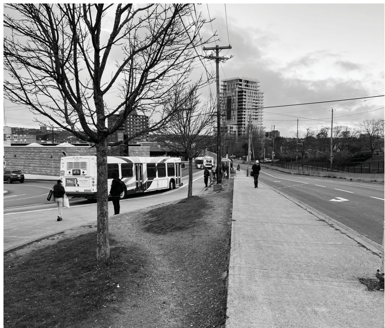
The 140-metre long sidewalk at Mumford Terminal Station
