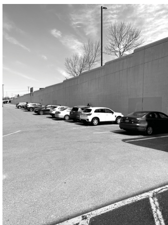
The site's six-metre retaining wall highlights the need for greater access universally designed public spaces.
