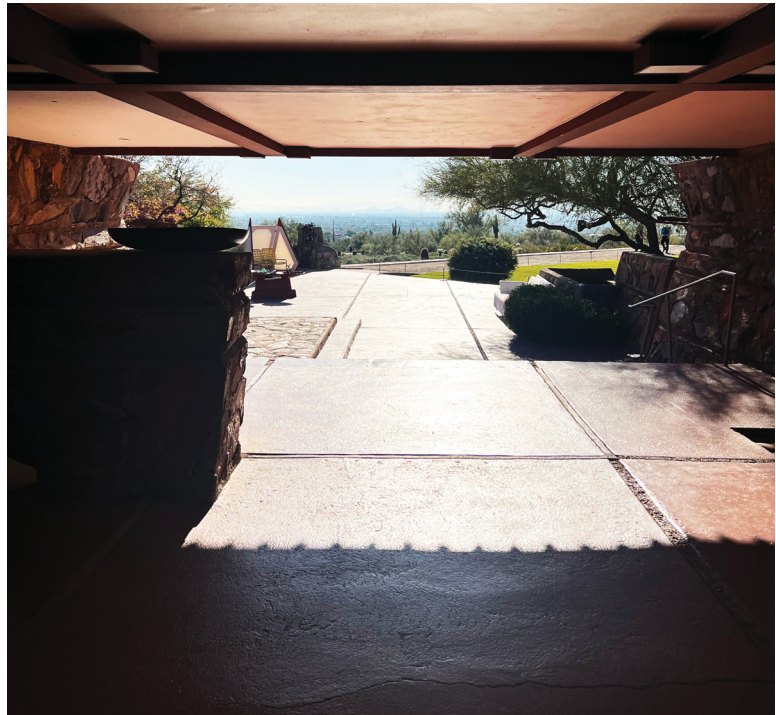
Passage between buildings causing the “Venturi effect” at Wright’s Taliesin West.
