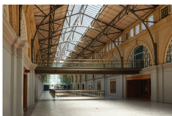
The reconstructed second floor of the Ferry Building (Schulenburg n.d.)
