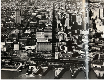
Ferry Building welcoming those to the redeveloping San Francisco, c. 1920; unknown photographer (Corbett 2010, 34)
