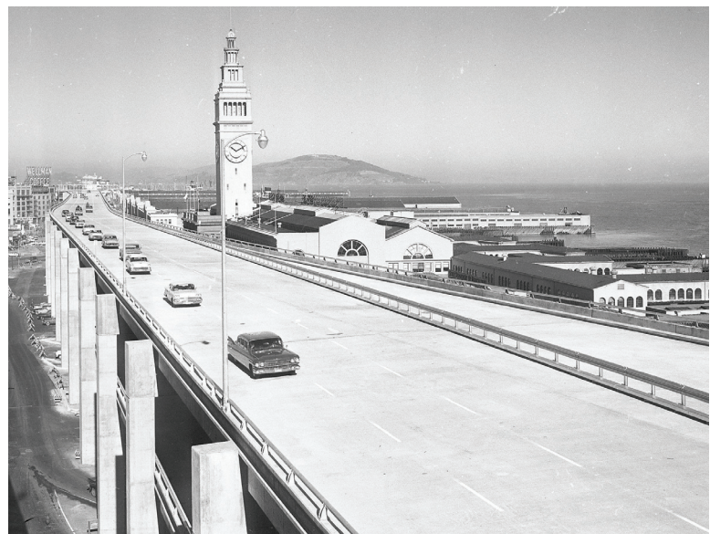
The Embarcadero freeway severing the Waterfront from the remainder of the city, n.d.; photograph by Ken Mclaughlin (Arredondo and Feldberg 2022)
