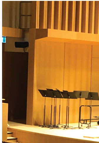
Cornice in the Strug Concert Hall, Halifax
