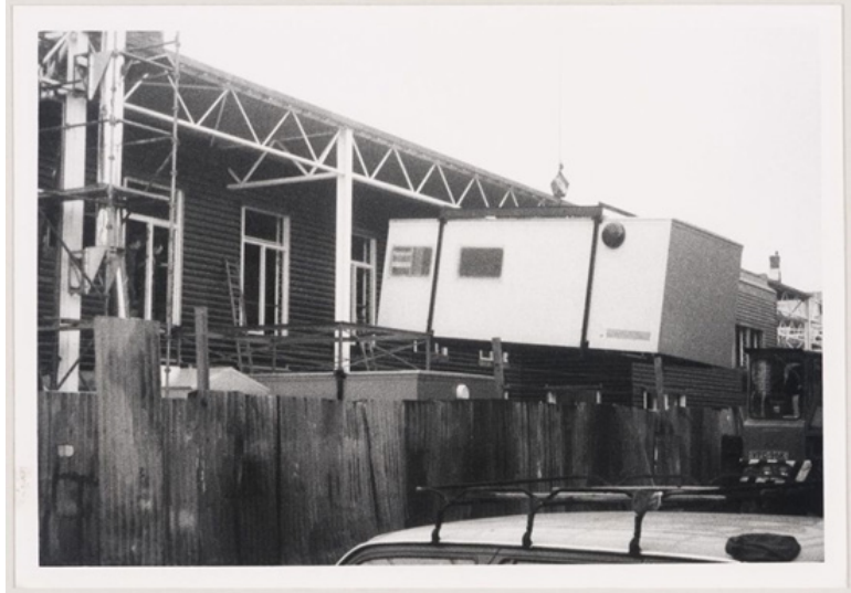
Cedric Price, Inter-Action Centre during construction, London, 1972 ("Hidden Architecture" 2017)
