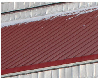
Figure 50: The existing red metal roofing, retained in the design proposal.
