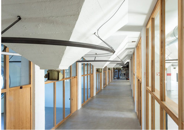
Figure 38: The bin hoppers of the Erlenmatt Silo feature as an architectural feature reminiscent of the building's past life (Harry Gugger Studio 2020).
