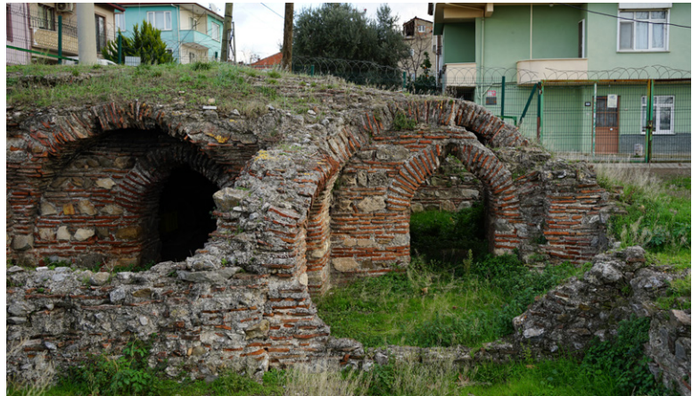
The Church on the corner is believed to be for burial. The Church is believed to be built here because many bodies were buried within the cavities of the Roman Theatre. The building materials of the church are believed to be re-used bricks and rubble spoliated from the Roman Theatre.
