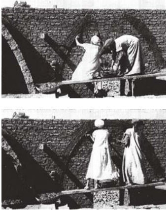
Traditional Egyptian construction using plaster to outline a parabola on the end wall (Fathy 1976, 245)
