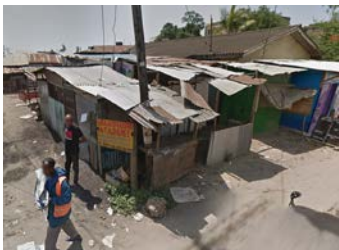
Non-durable metal sheet housing in Chaani, Mombasa (Google Street View n.d.).
