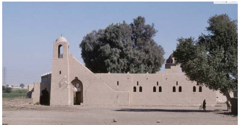
New Gourna Mosque, built using traditional materials and construction methods (Blair 1978).
