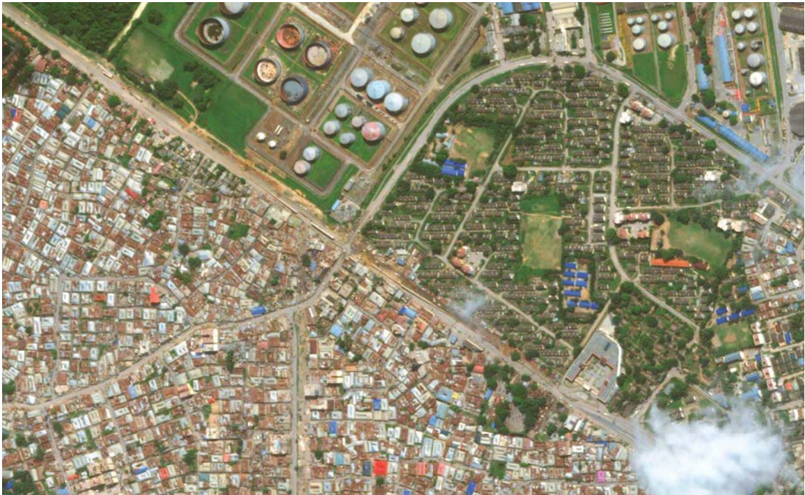
Mombasa's airport road splits an informal settlement from a developed neighbourhood and a petroleum refinery. Many informal settlement remain trapped by such roads, leaving little room for lateral growth (Google Earth n.d.)
