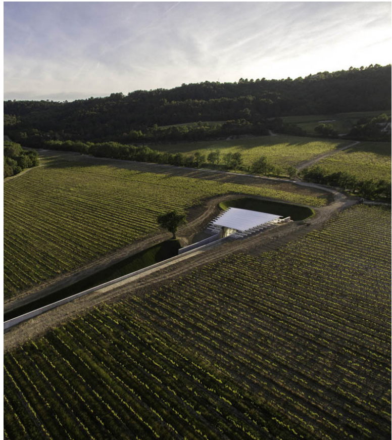
Renzo Piano Building Workshop, Chateau La Coste Art Gallery & Barrel Storage. The building is sunk into the ground to limit the shadows cast on the vineyard. The roof structure follows the same spacing as the vines (RPBW 2009).
