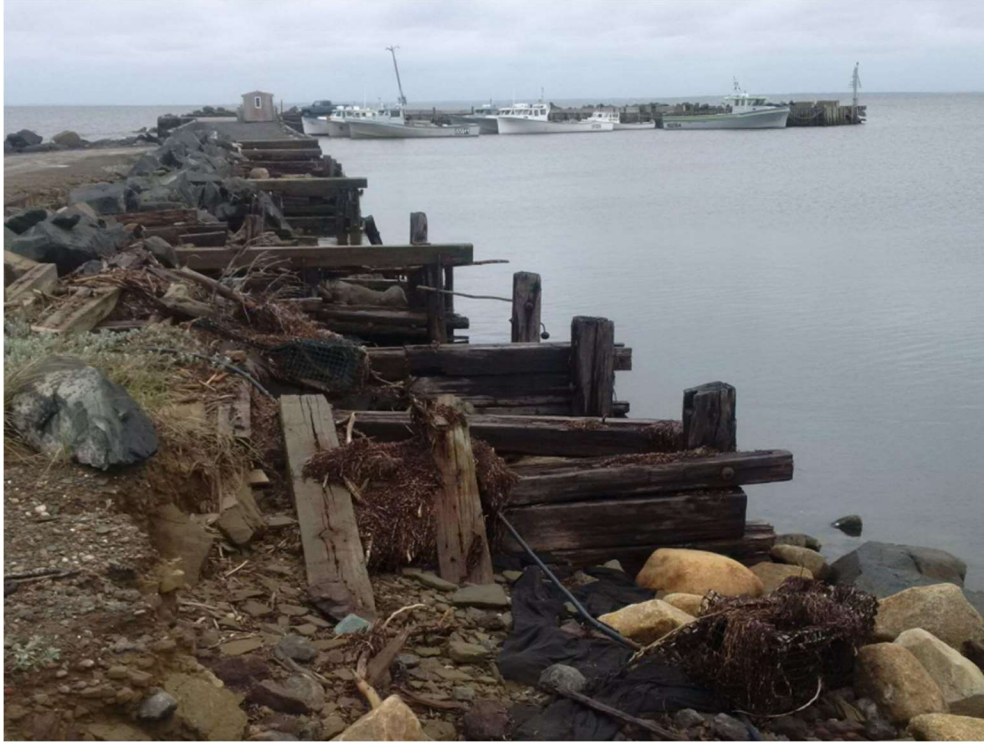
Figure 2 Non-Core Wharf at Esgenoôpetitj, New Brunswick (McDonald, 2019)
