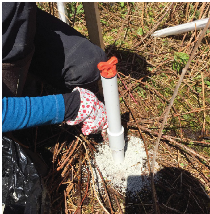
Figure 4. Monitoring well installation in focused study plot
