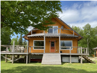
Terra Nova cottages
