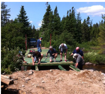
Terra Nova residents working together to repair cabin access bridge
