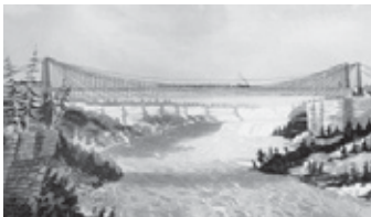
The Niagara River Suspension Bridge which was completed in 1855 (Griggs 2016).
