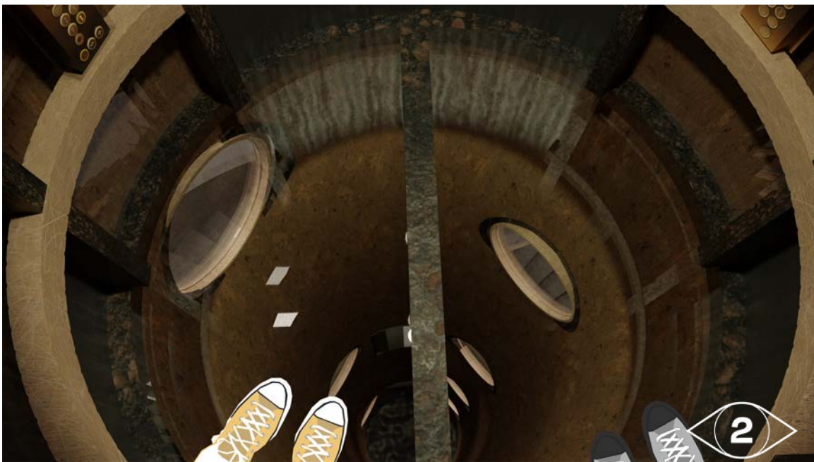
Interior perspective of the elevator inside of the penstock, looking down towards the Turbine Deck.
