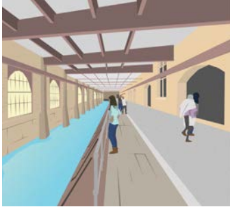
Interior perspective of the Rankine Generating Station showing fore-bay which feeds the penstocks. Key features include the grating that protects the turbines from large debris and the steel and masonry construction of the structure.
