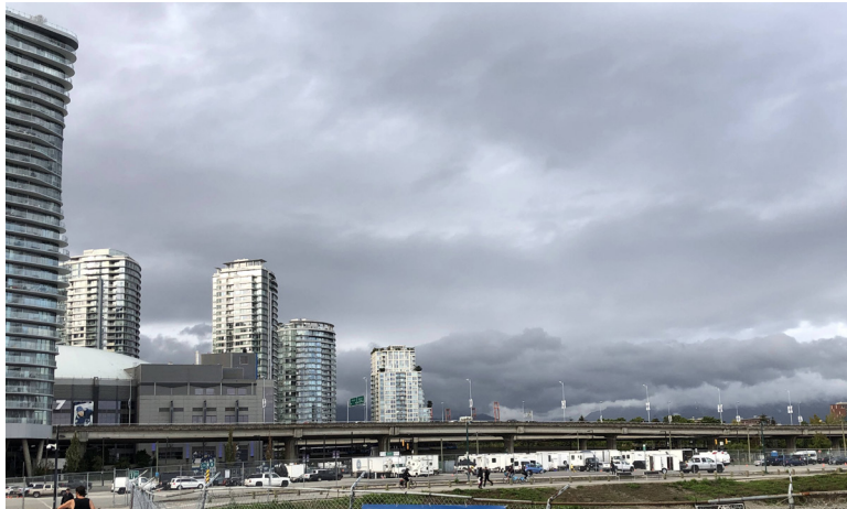
Fig. 17. Looking north toward the viaducts, showing the abrupt end to the high-rise buildings moving eastward
