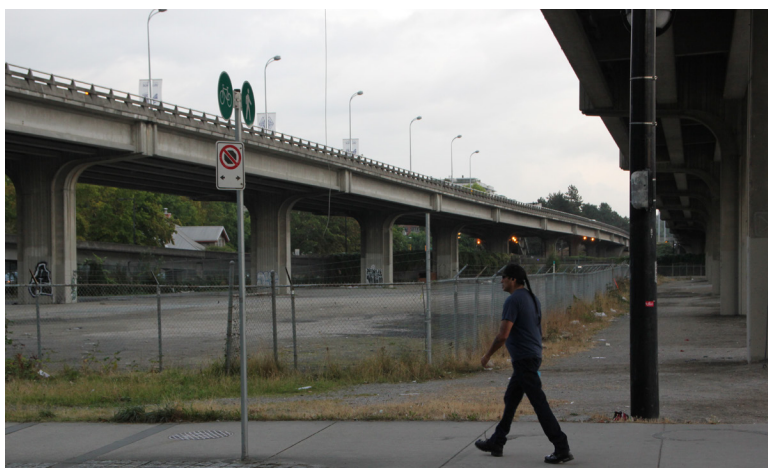
Fig. 18. Looking eastward between the two viaducts at grade, showing a vast fenced-in area void of programming
