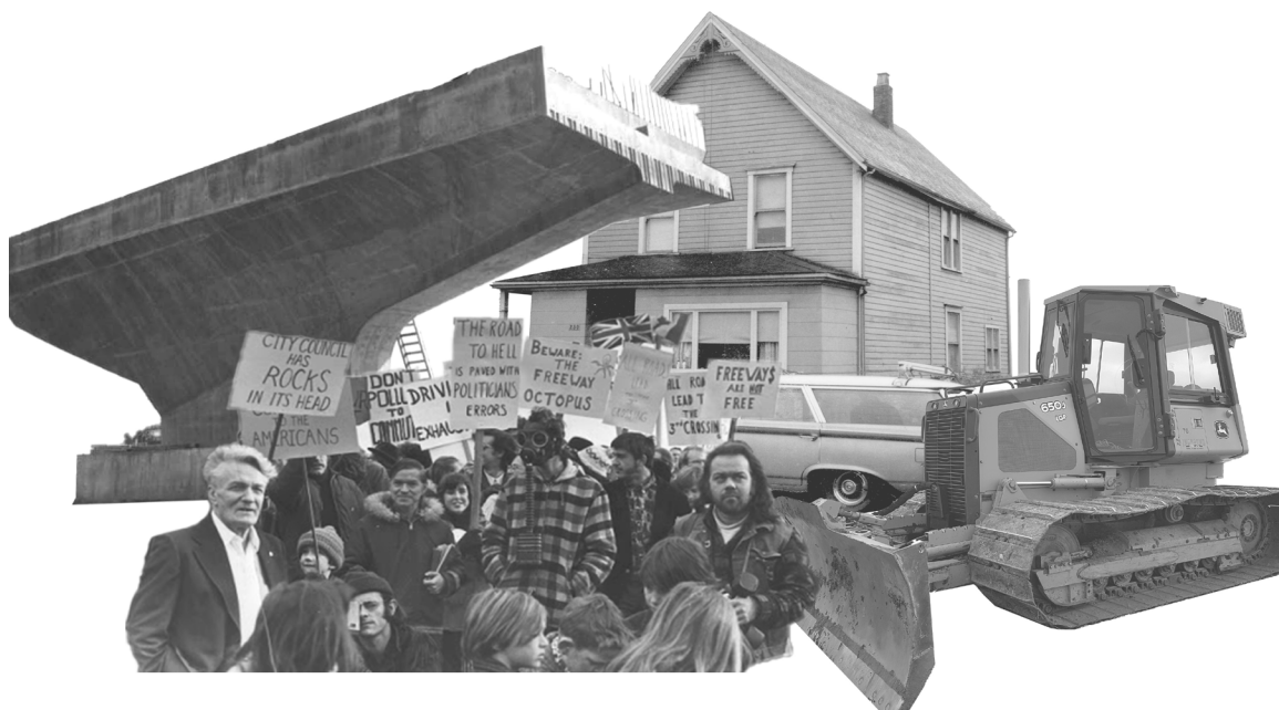
Fig. 8. In the early 1970s the new viaducts were built to replace the original, displacing entire communities in their wake. Community members continued to push back, including an active demonstration which blocked the mayor’s limousine from crossing the viaducts on opening day.
