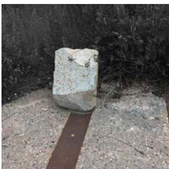
Concrete surface with steel tracks.
