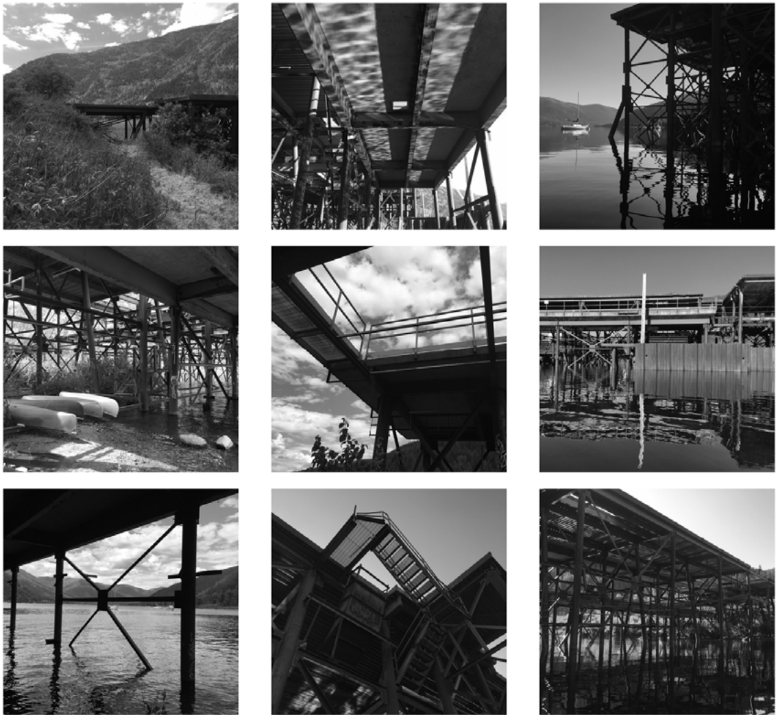
Images of the existing pier's structure.
