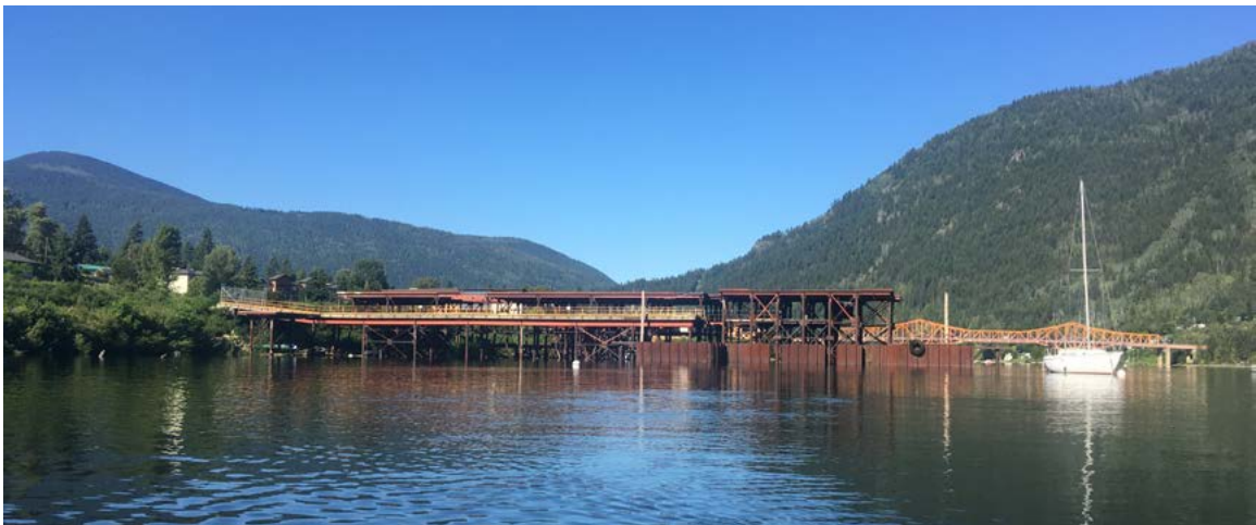
Existing pier extending out into the West Arm of Kootenay Lake.
