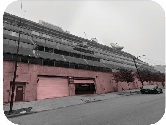
South-east facade of CBC Headquarters
