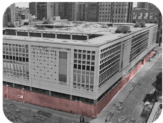
North-east and north-west facades of the Canada Post building
