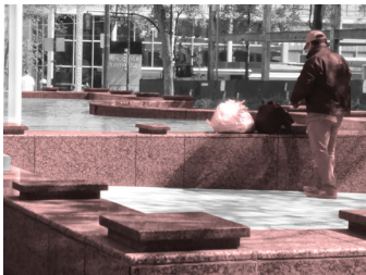
Defensively designed fountain ledge deters skateboarding and sleeping. Photo taken downtown Vancouver outside an office building.
