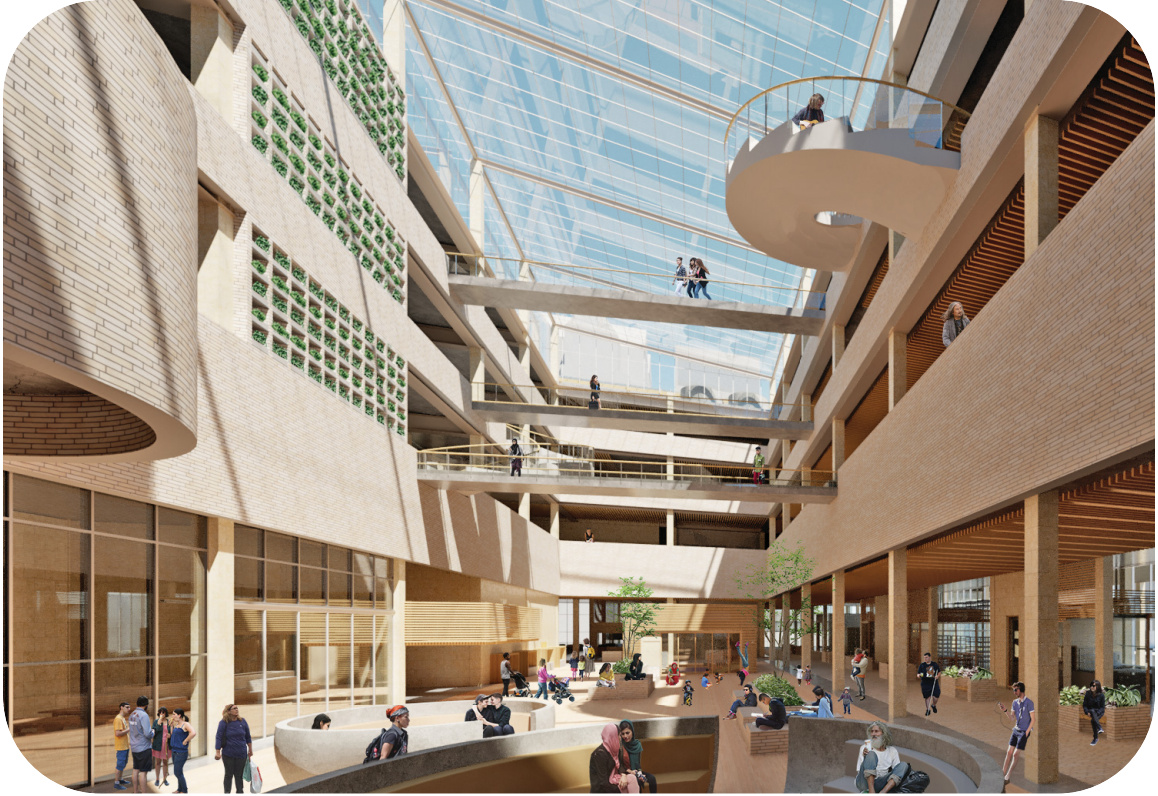
View of the long central atrium in the building looking to the north-east.
