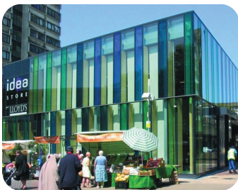
Idea Store on Chrisp Street, London, UK; designed by Adjaye and Associates (Adjaye and Associates 2020)
