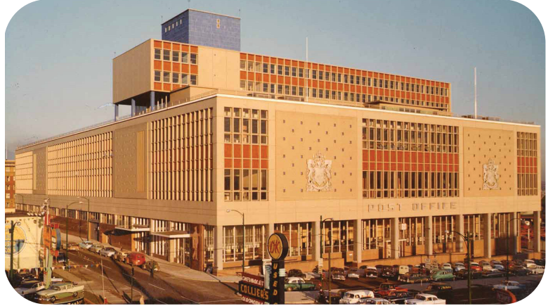
Vancouver Main Post Office as constructed in 1953 (Landauer 1960)
