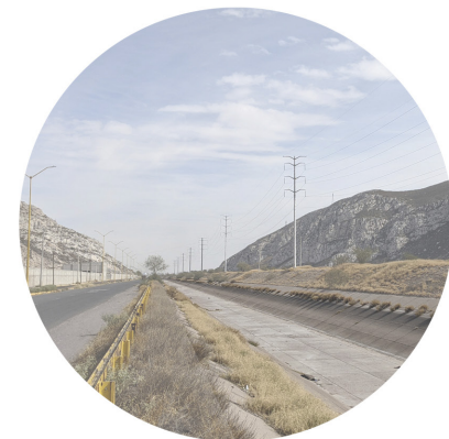
8 - concrete-lined Canal de Sacramento
