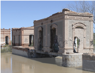
Brick masonry is also a commonly used material in the Laguna.
