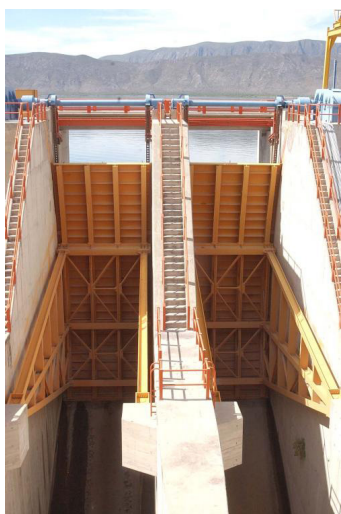
Photograph of the Francisco Zarco Dam's gates that control the Nazas River. (Yomontaño-W-S 2008).
