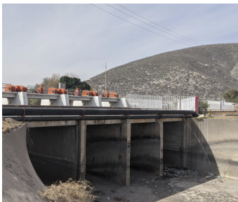
1 - San Fernando Derivation Dam. (Photograph by author, 2021).
