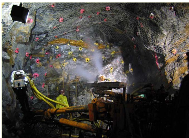
Figure 2- 3: Drill and blast tunnel (civildigital.com)
