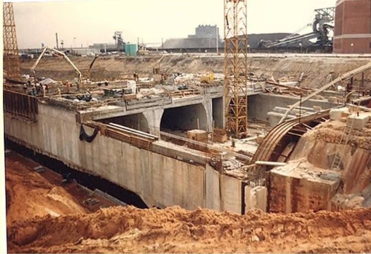
Figure 2- 2: Cut and cover top-down tunnel (civildigital.com)
