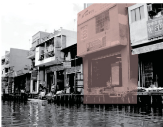
A study of existing adaptations to vernacular building strategies. Corrugated metal wall material (above) and stilted structure with veranda access to water (below).
