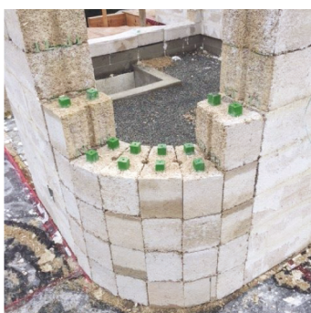
Figure 40: JustBio Fibre Blocks used to create curved walls (JustBio Fibre Structural Solutions 2017)
