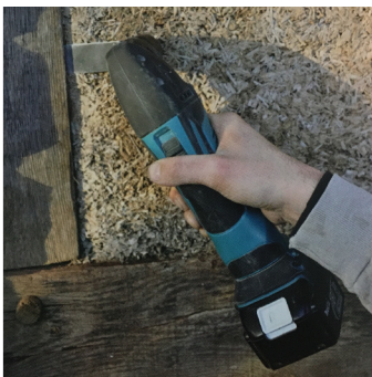
Figure 59: A multi-tool is useful for carving and shaping hempcrete. (Stanwix and Sparrow 2014, 106)
