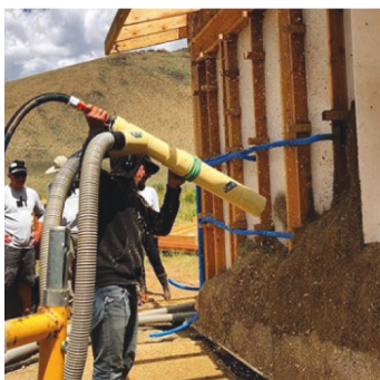
Figure 50: Instalng hemcrete via spray applied (Hempitecture 2019)
