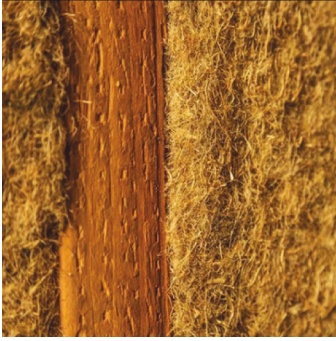
Figure 54: Closeup of the fibres in the hemp quilt product. Note the tight fit of the batts into the stud cavity.
