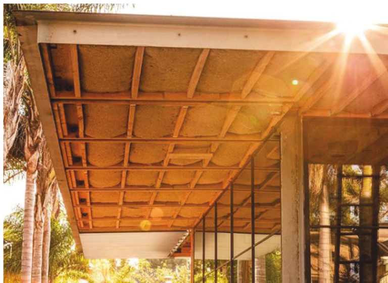
Figure 10: HempWool insulation installed in a roof joist (Hempitecture 2020a)
