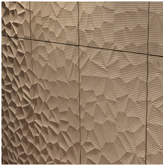
Herzog & de Meuron, edge conditions of custom acoustic CNC wall panels in the Elb Philharmonie, Hamburg, 2007-2017
