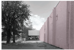
Connectors between the Fielding, Common school and the Junior High Building
