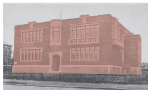
Bloomfield Common School Architect: William Fraser Constructed in the year 1919 (front facade facing Robie Street)
