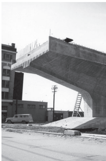
View of the construction of the Georgia Viaduct, 1970; photograph by Vancouver Engineering Services, from the Vancouver Heritage Foundation.
