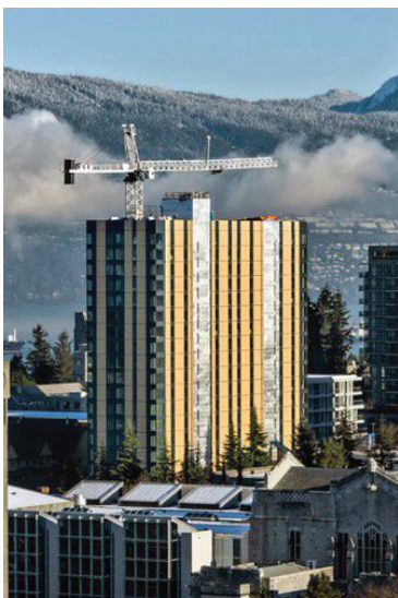
Brock Commons, 18-story wood building in Vancouver; photograph from Lara Shecter, 2018, https://www.naturallywood.com/BCT-performance .
