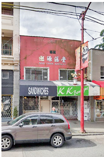
Soo Yuen Society facade; image from Google Maps.
