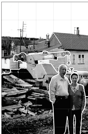
Collage of the Strathcona Demolition.
