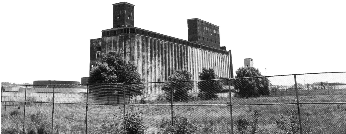
“The Port of New York Authority Grain Terminal” has been left abandoned and decaying since the late 20th century. Old industrial buildings are scattered in what used to be the busiest industrial port in North America.
