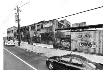
Vacant industrial building is common in Red Hook (Google Maps 2018)
