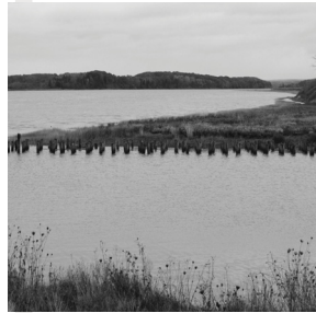
WOODEN PIER OF FORMER SHIPPING PORT
