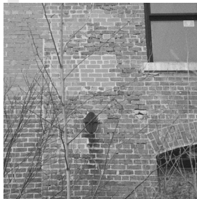
INTERNAL STRUCTURE EXPOSED
