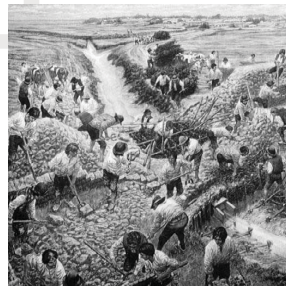
DIKES BEING BUILT 1700
