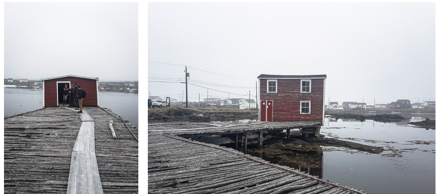
The Dwyer Premises in Tilting, Fogo Island consists of a house and outbuildings associated with the family-based inshore fishery. (Photos from M1 studio trip in May, 2017).
