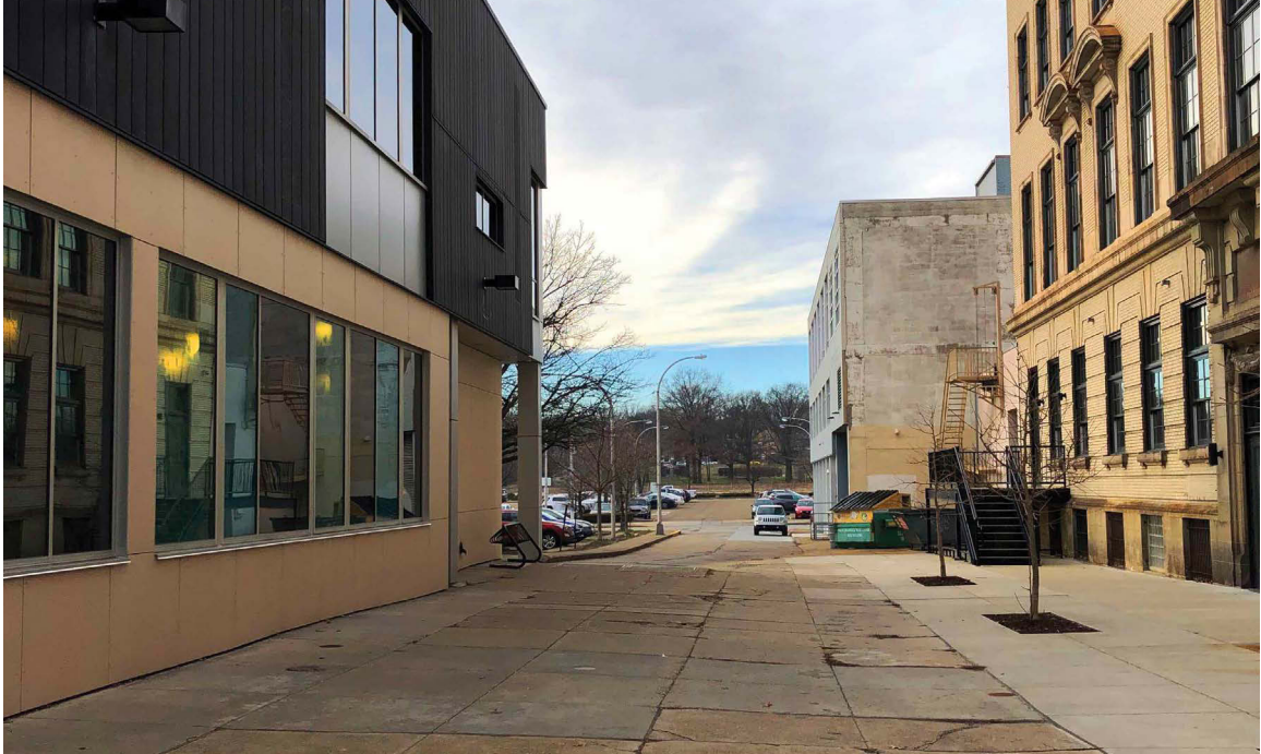
View looking northeast towards the site from the East Liberty Carnegie Library and the Ace Hotel. The Cathedral of Hope is directly behind the view.
