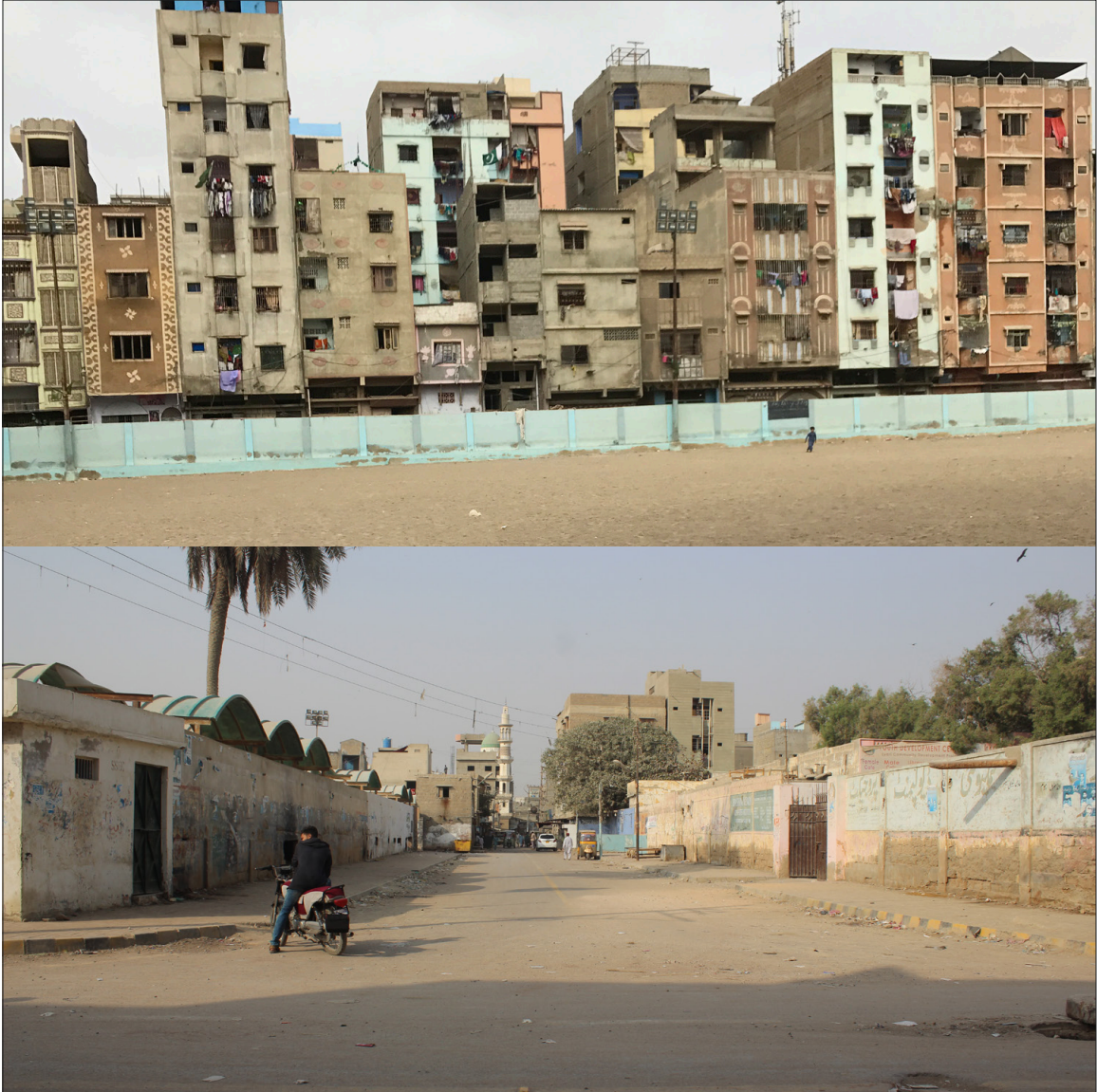
Building traditions and materials in Lyari. Concrete block houses painted in colours and cinder blocks and boundary walls enclosing public spaces.
