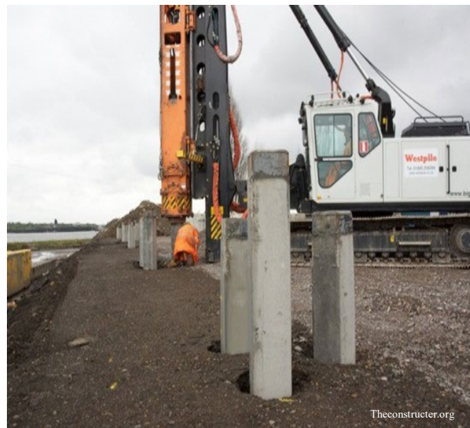
Figure 2. 6 Driven Precast Concrete Piles (The constructor website)
