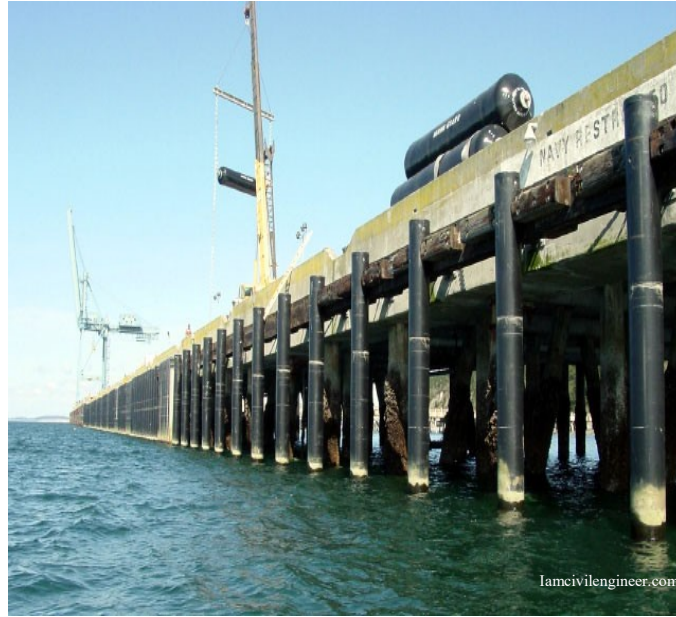
Figure 2. 3 Fender Piles (I am civil engineer website)
