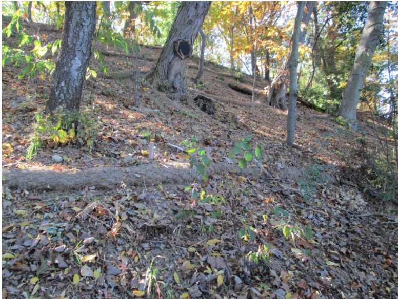
Figure 6.8.46: Slope restoration near Fresh Pond Golf Course. Saulnier, October 20, 2013.
