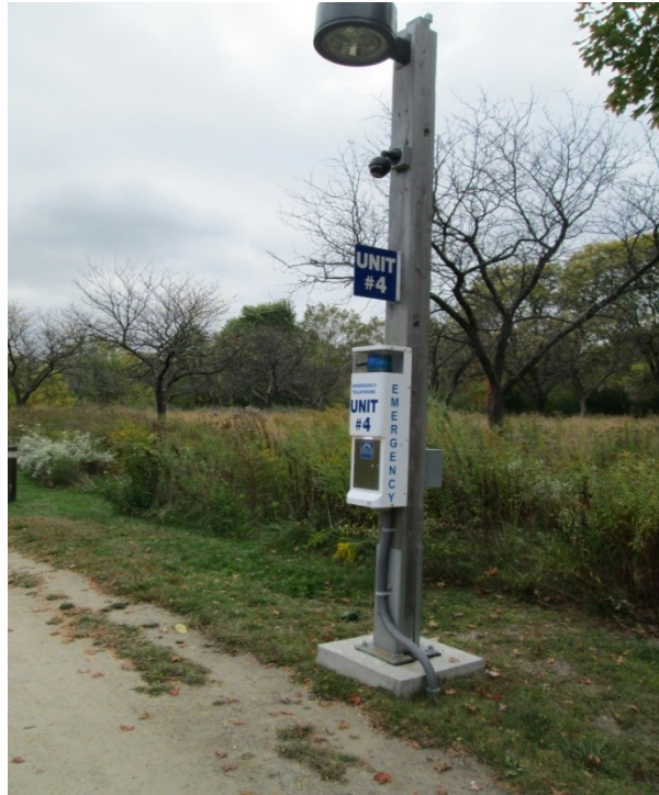
Figure 6.8.9: New lighting and emergency phone located throughout the path towards the T-Station. Saulnier, October 17, 2013.
