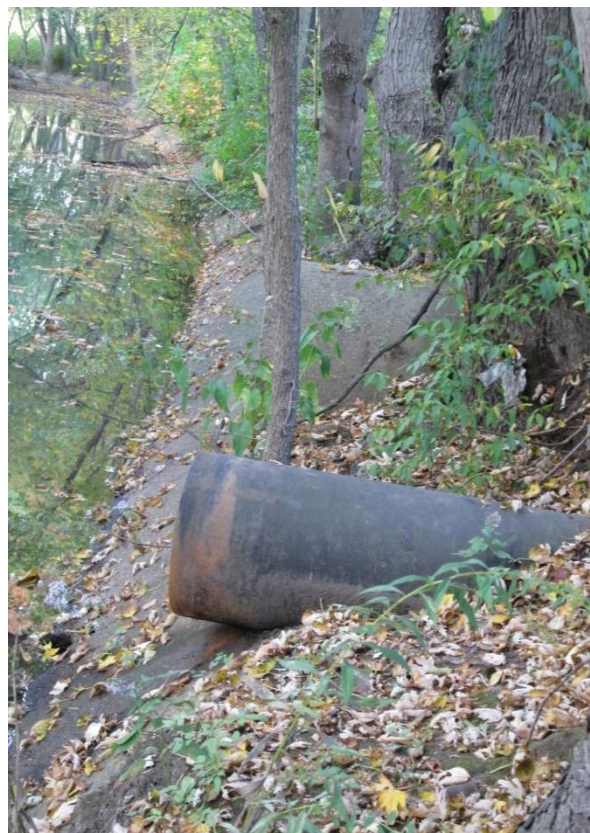
Figure 6.8.35: Several stormwater pipes are located along the Alewife Brook. Saulnier, October 17, 2013.
