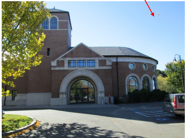
Figure 6.8.42: Fresh Pond Water Treatment plant. Saulnier, October 20, 2013.
