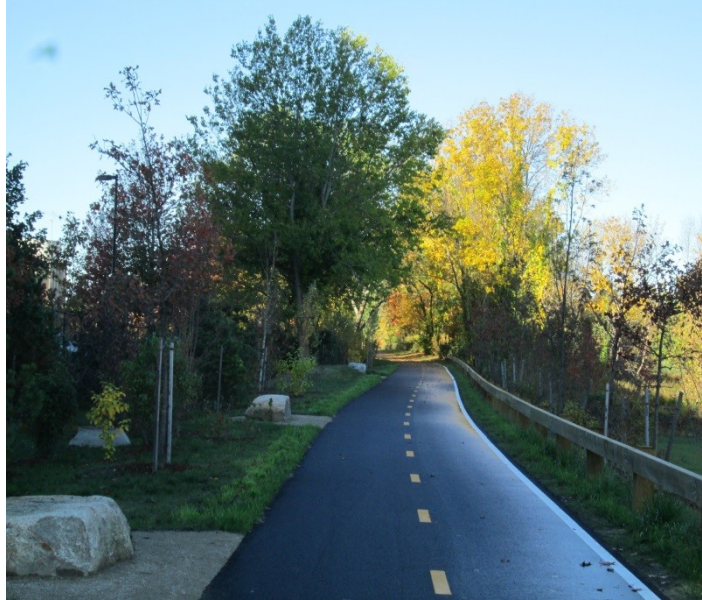
Figure 6.8.19: Newly paved bikeway at the Stormwater Wetland. Saulnier, October 17, 2013
