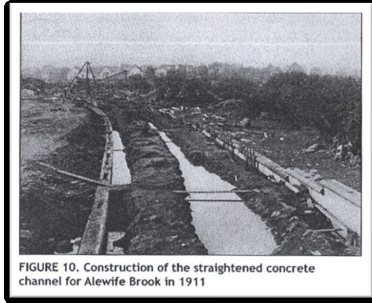
Figure 3.3.1: The Alewife Brook in 1911, straightened into a concrete channel (TBG, 2003).
