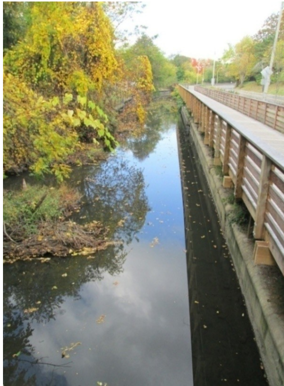
Figure 6.8.32: New boardwalk on the South side of Alewife Brook. Saulnier, October 17, 2013.
