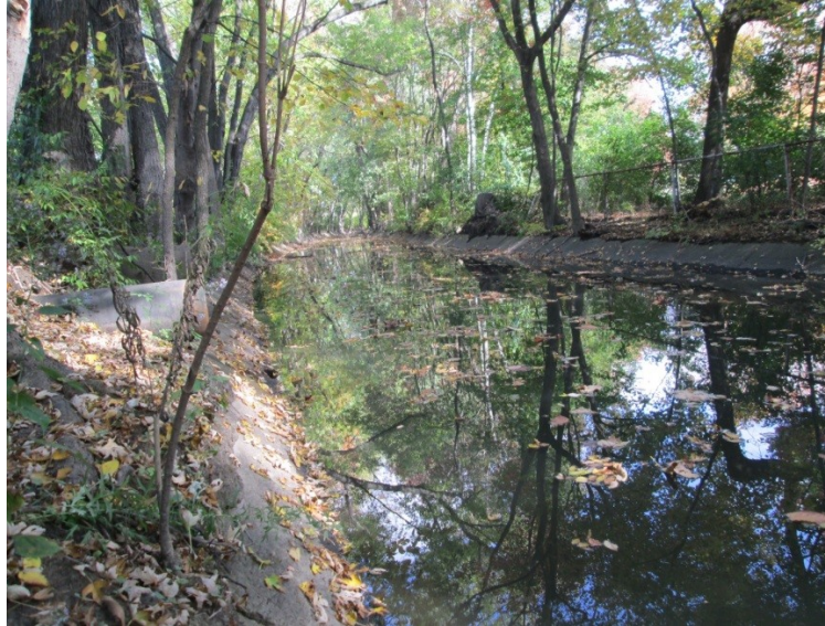
Figure 6.8.34: Alewife Brook with concrete banks. Saulnier, October 17, 2013.
