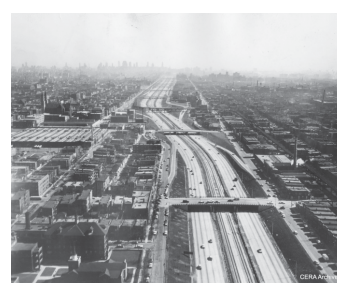
Aerial View of Eisenhower Expressway (CERA Chicago)
