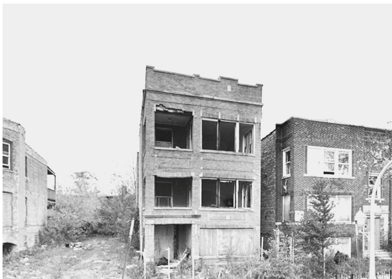
Urban Decay, West Garfield Park (Google Maps).
