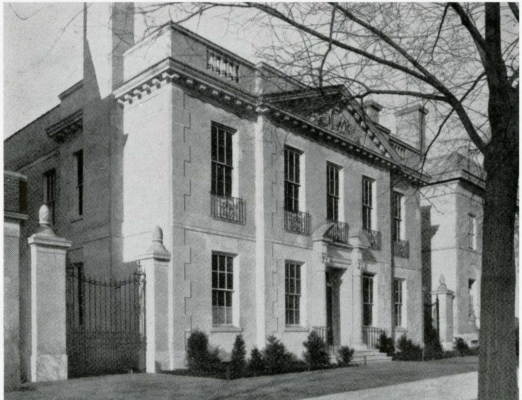
HEAD OFFICE BUILDING FOR PROVINCIAL PAPER LIMITED, UNIVERSITY AVE., TORONTO MARANI AND LAWSON, ARCHITECTS
