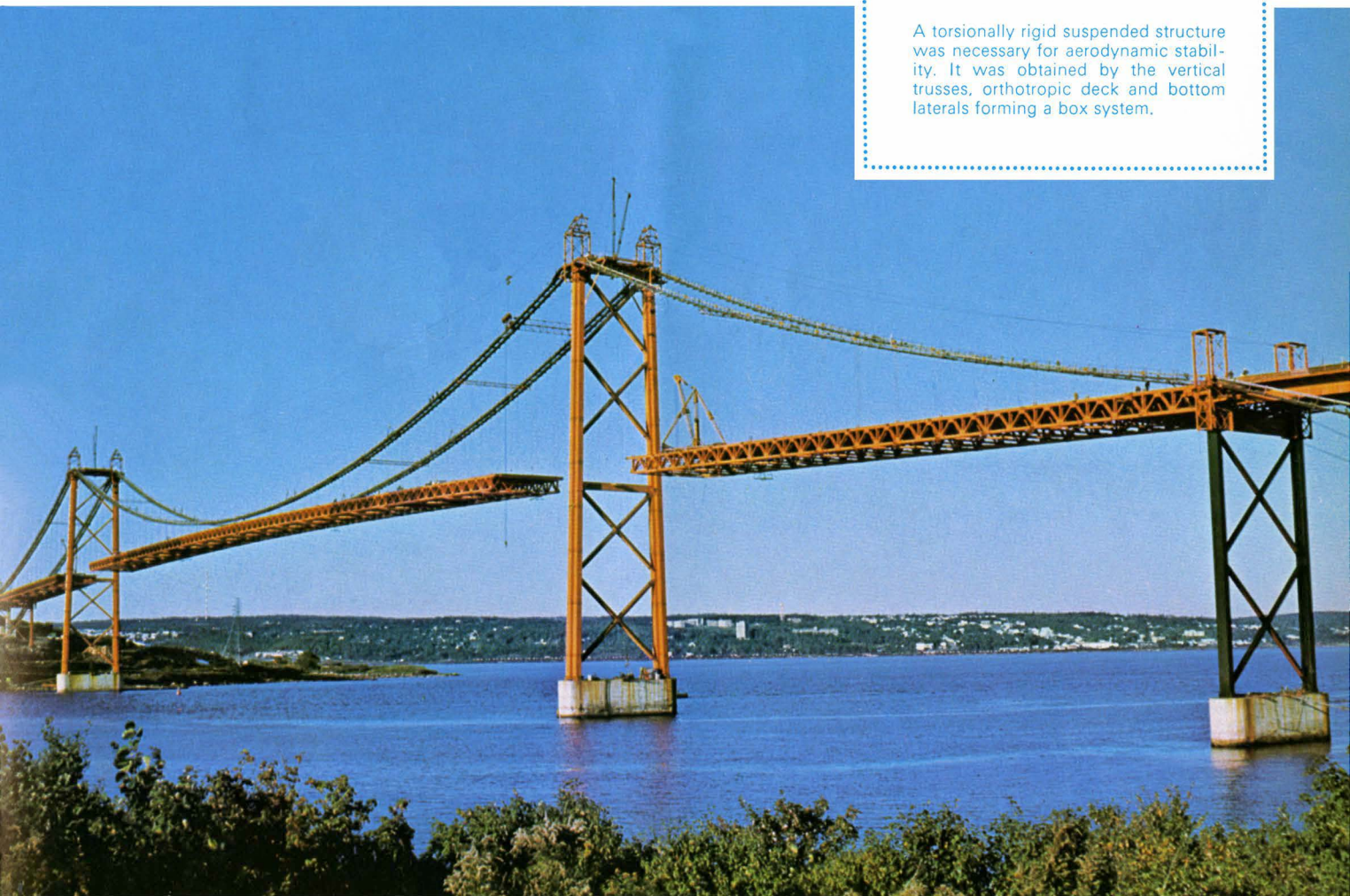
Halifax A. Murray MacKay Bridge nearing completion
