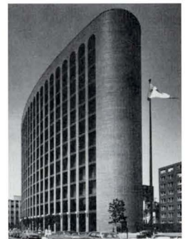
PSA office building
