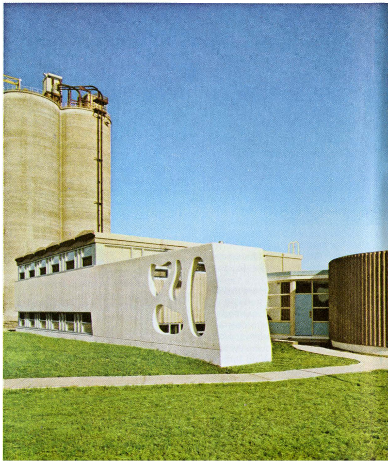
5 Decorative concrete wall at Canada Cement plant near Saskatoon.
