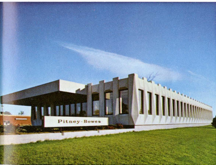
7 Pitney-Bowes Building, Ottawa, Ont.
