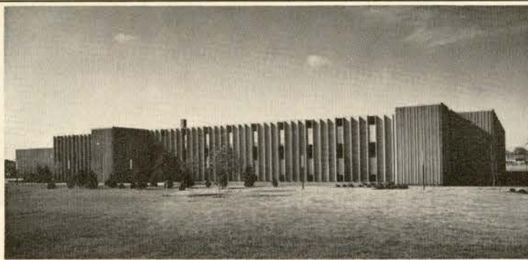
Zion Heights Junior High School, North York. Arch: James A. Murray, Toronto. Eng: G. Granek & Assoc. Don Mills.
