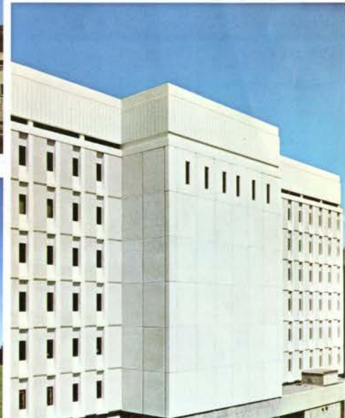
9 Pathology Institute Building, Halifax, N.S.
