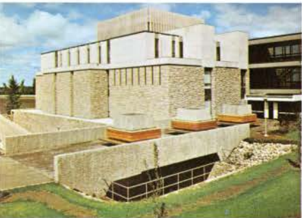
3 Precast concrete pedestrian bridge at University of Saskatchewan.
