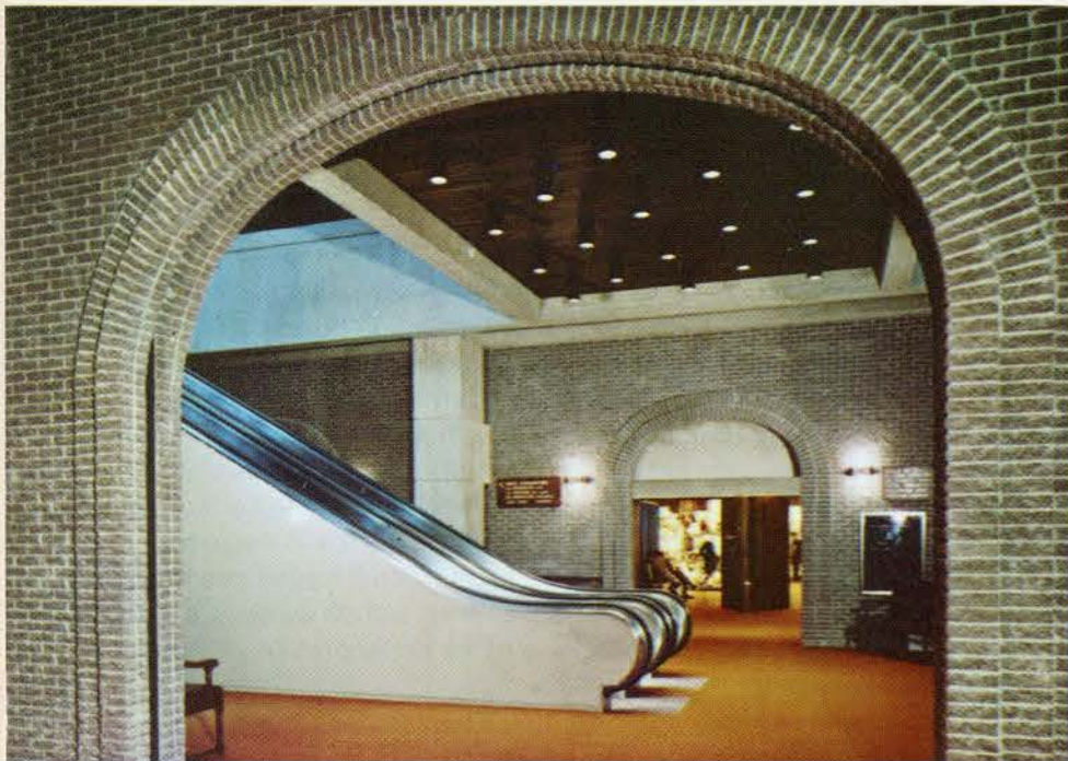
Many interior walls feature coloured and textured concrete masonry units.
