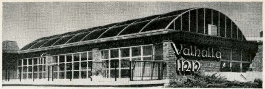
Valhalla Inn, Toronto 33' x 73' barrel-vault Plexiglas cover. Plexiglas color 2412, Bronze Formed by English Plastics Ltd., Brampton. Designed and erected by Ickes-Braun Glasshouses of Canada, Beamsville, Ont.
