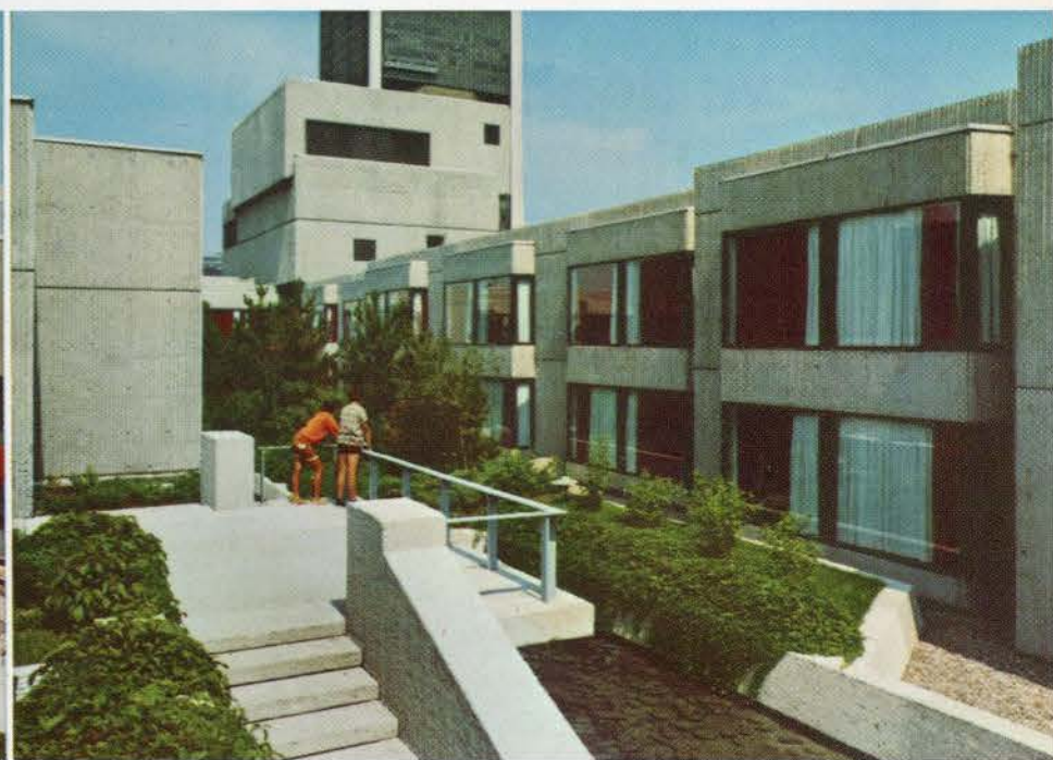
A section of the roof-garden terrace adjoining the two-storey hotel.
