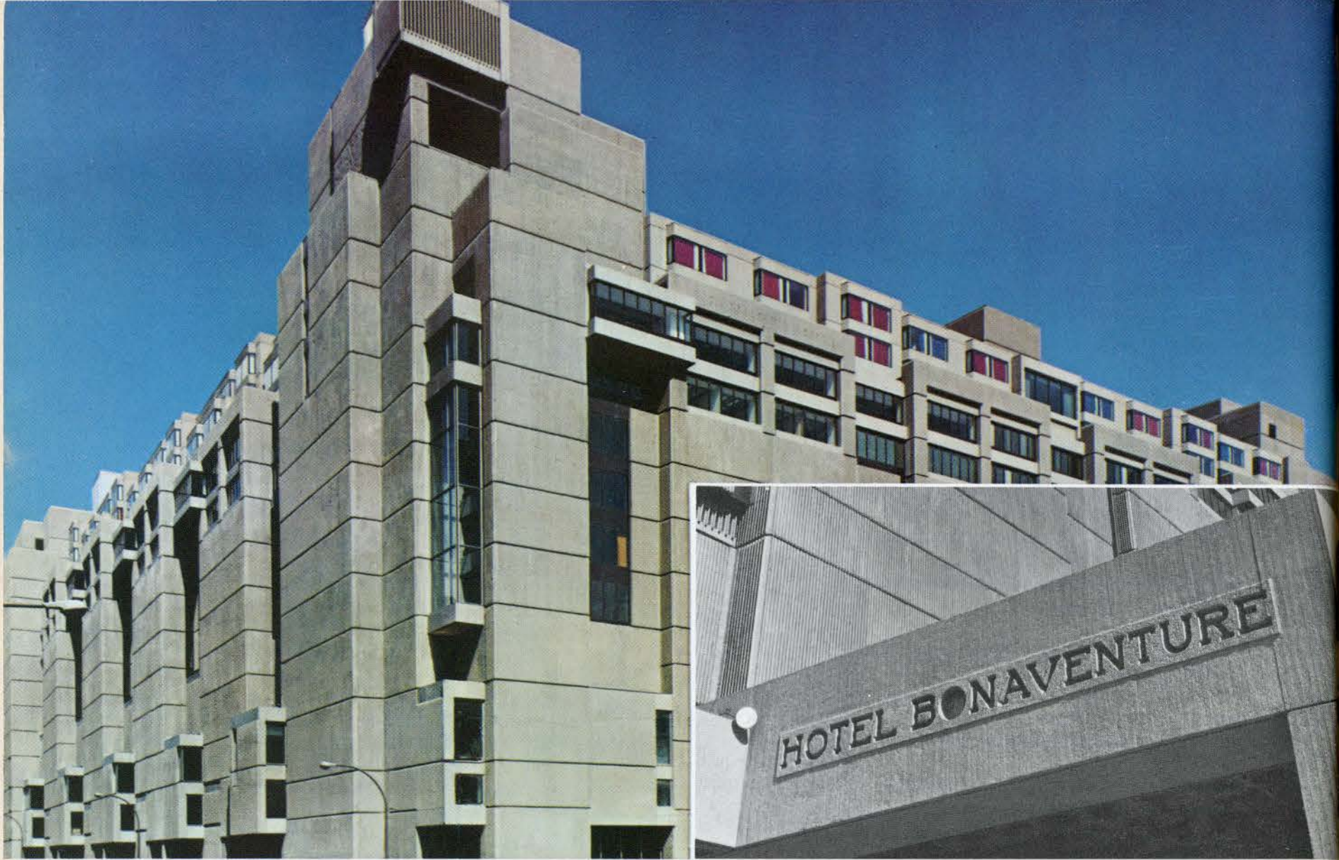
The exterior of this mammoth trade centre in downtown Montreal features exposed aggregate concrete walls having a vertically fluted pattern.
