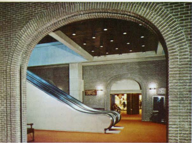
Many interior walls feature coloured and textured concrete masonry units.
