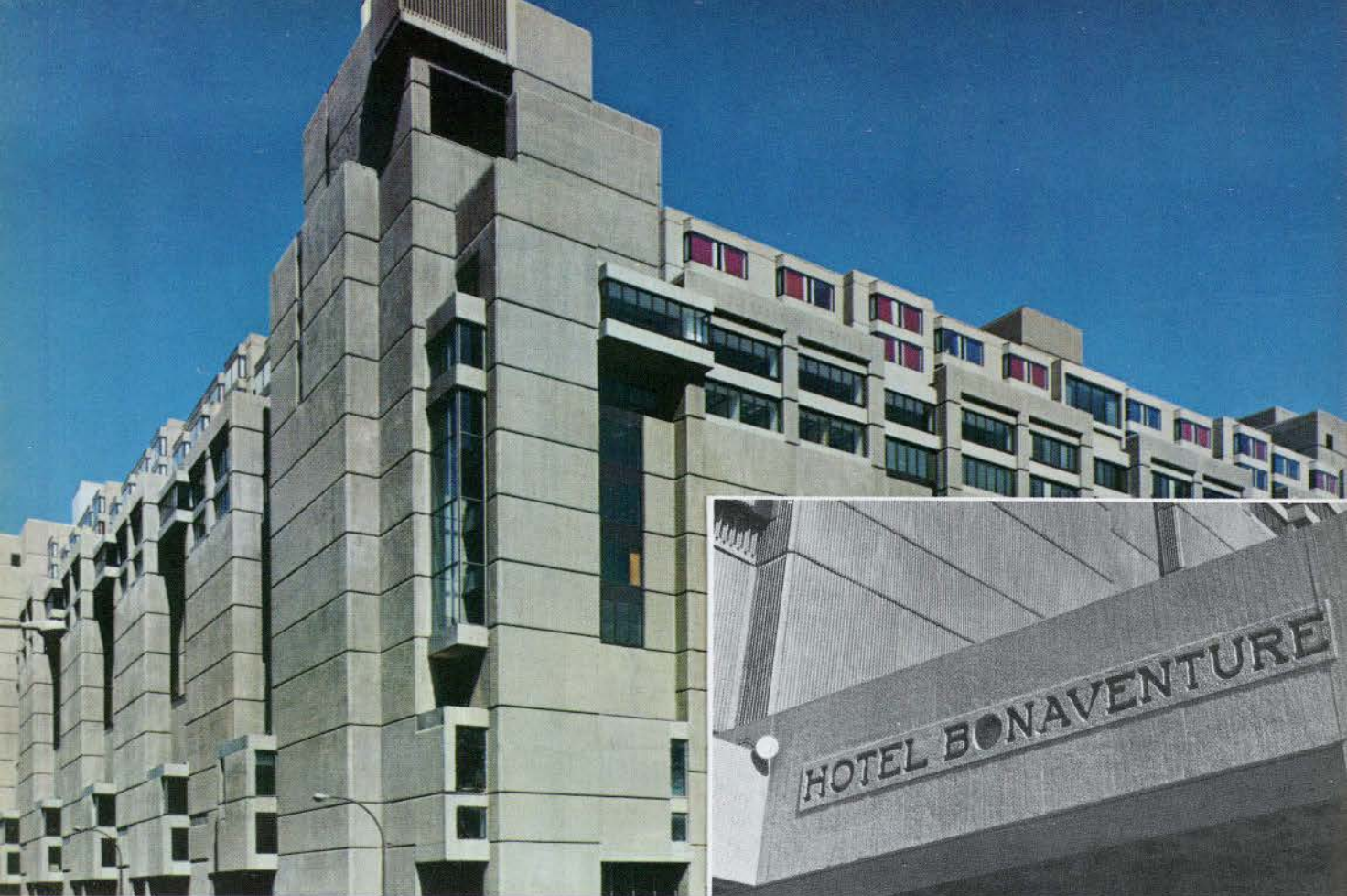
The exterior of this mammoth trade centre in downtown Montreal features exposed aggregate concrete walls having a vertically fluted pattern.
