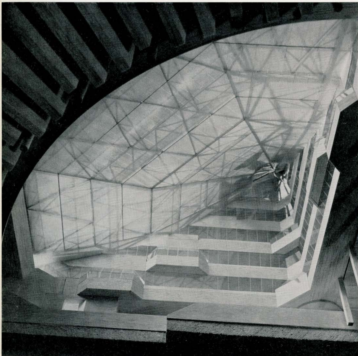
Cambridge History Faculty, 1964-68 (under construction), James Stirling Architect
